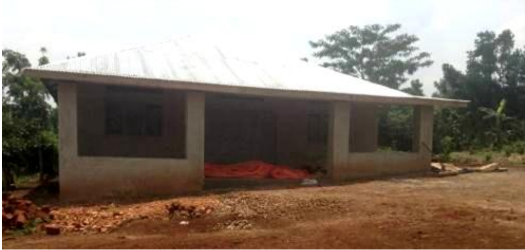
Above is the store that holds the six silos
